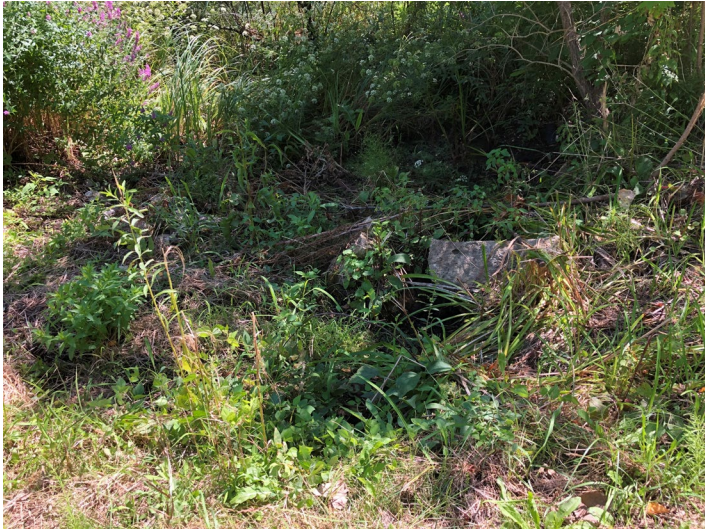
Photo 5: Existing stormwater culvert
