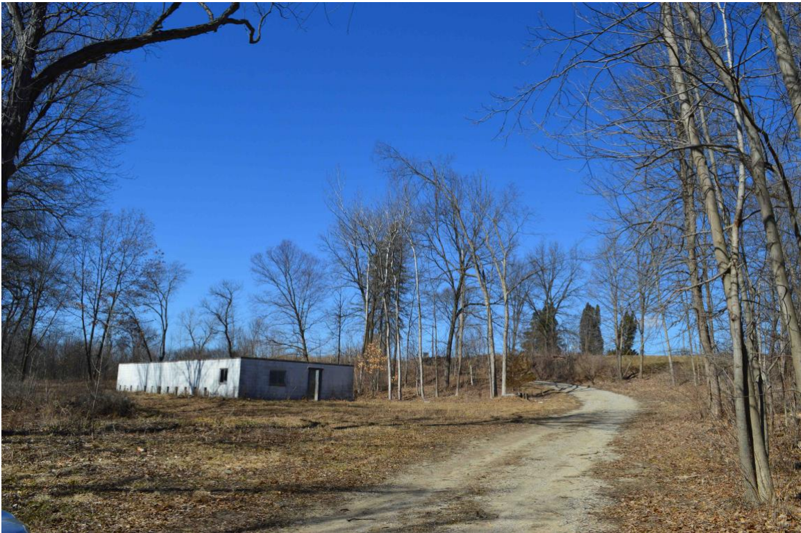
Photo 2: Restroom, facing north.
