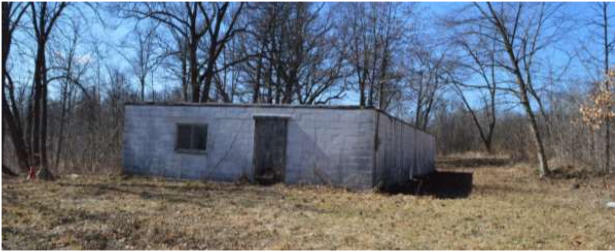
Photo 5 – Only remaining above-ground structure on parcel, former campground office, March 2021
